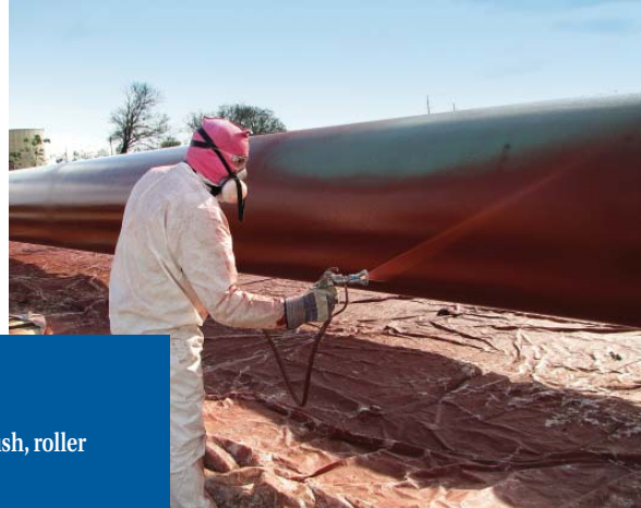
Protal ARO being spray applied.
